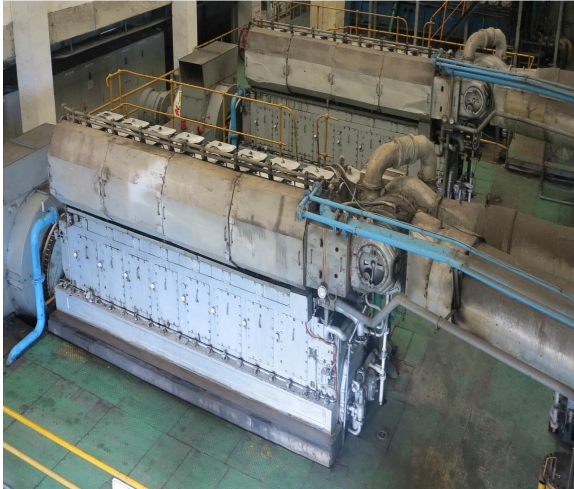
Two (2) 4.2 MW Mirrlees Blackstone bunker engine
