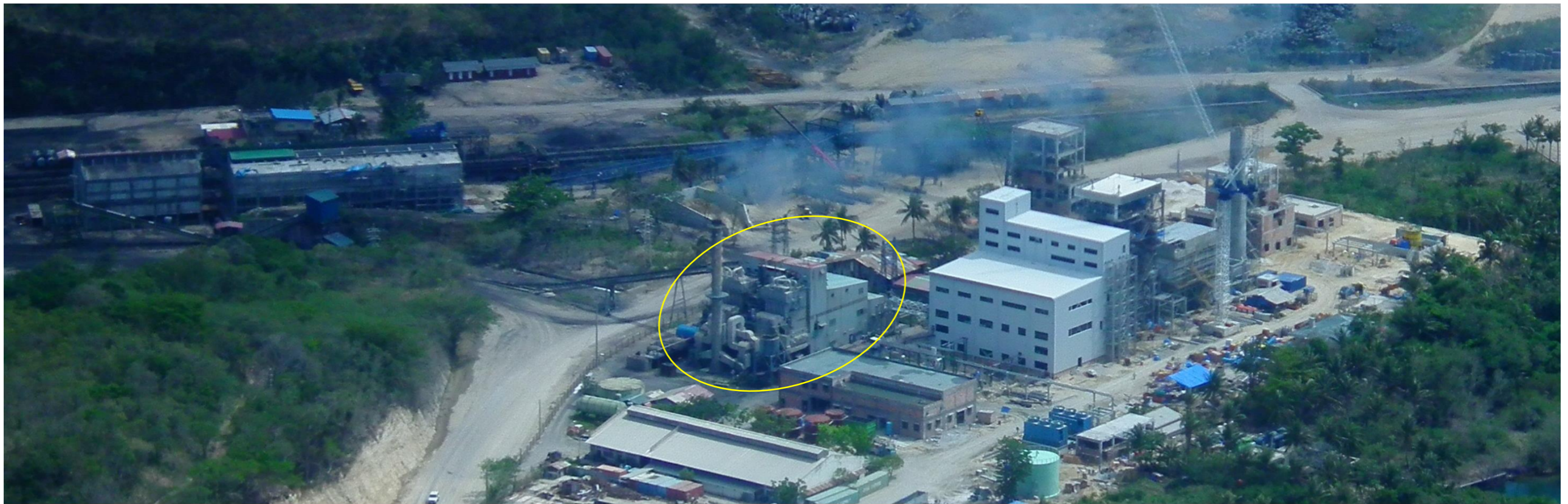
Additional One (1) unit 15 MW coal-fired power plant
