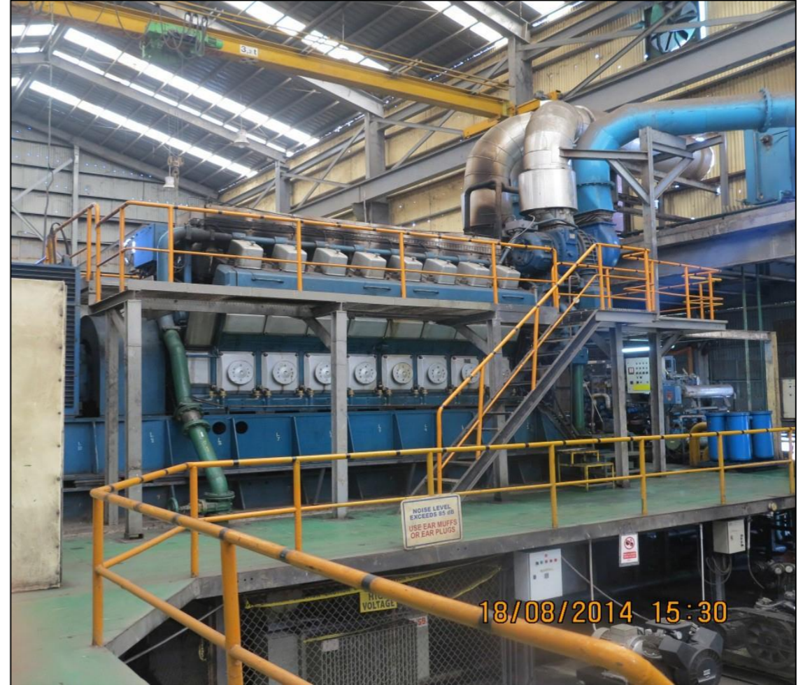
One (1) 5.7 MW Wartsila bunker engine
