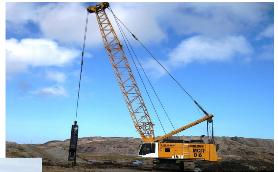
Grab Crane, Leibherr Two (2) units
